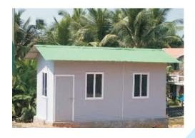
The porta cabin fabrications pipe structure purlins & grid Roofing sheet, Wall use cement panel & Puff Panel, door & windows.
